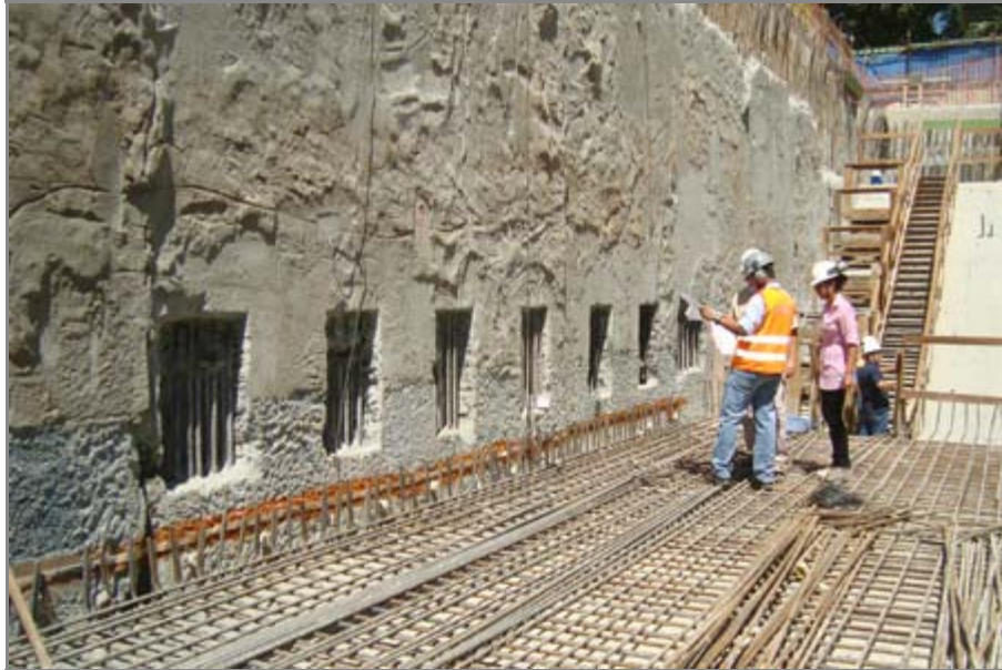
View of the Nossa Senhora da Paz station at Leblon; PENEBAR SW-55 was used for the concrete joints and PENETRON for the bridge.
