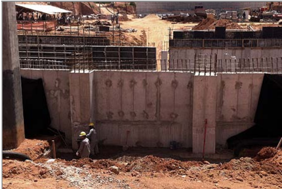
View of the concrete wall treated with PENETRON and PENECEM MORTAR.
