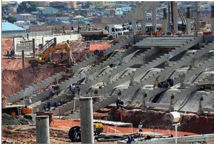
PENETRON ADMIX-treated concrete at Arena Corinthians.
