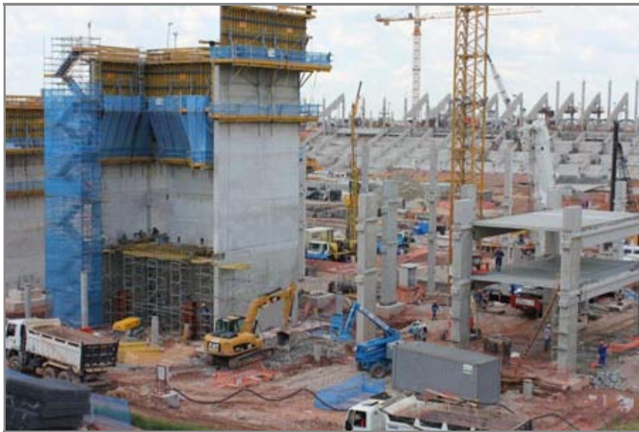
Arena Corinthians under construction.
