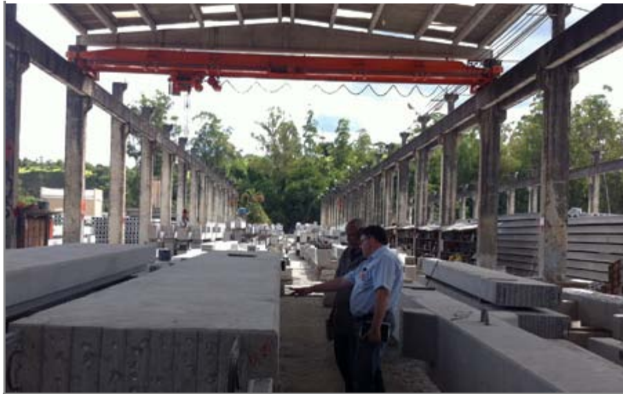
Close-up of PENETRON ADMIX-treated concrete beams for Mineirão Stadium.
