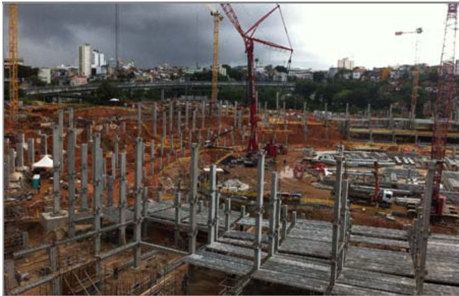
Fonte Nova Stadium under construction.
