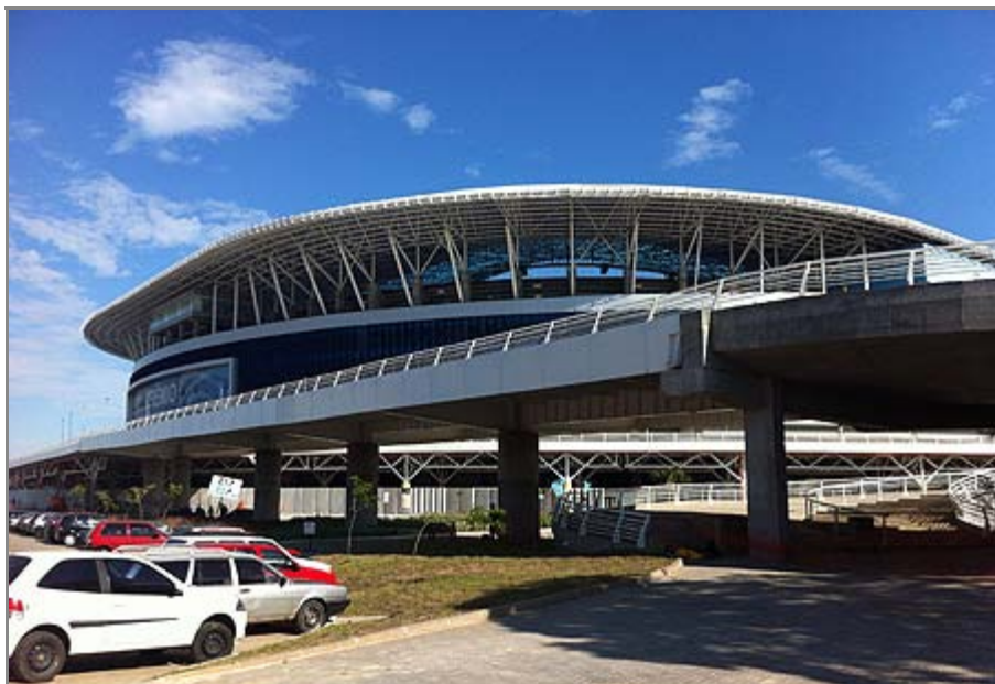
Side view of the PENETRON ADMIX-treated ramp.
