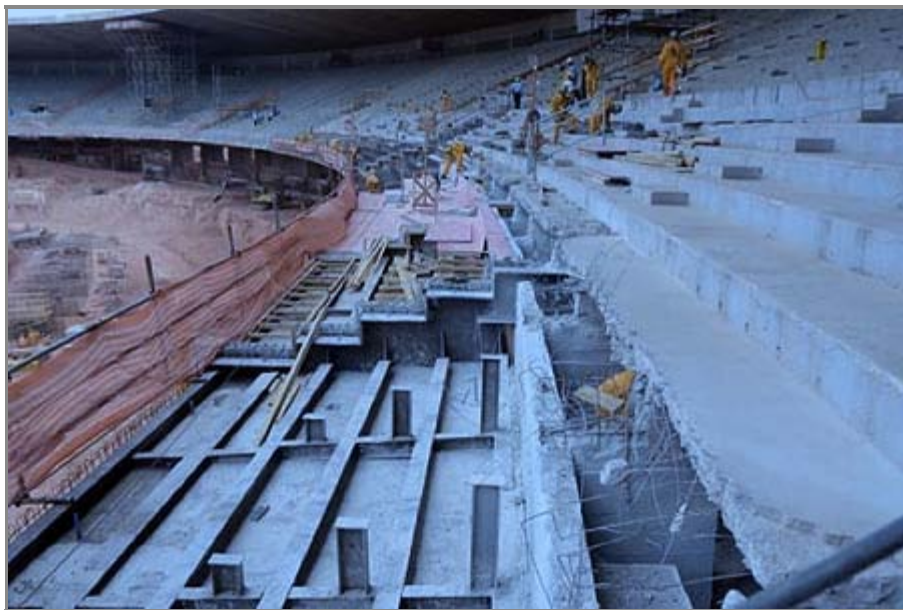
The grandstand under construction.
