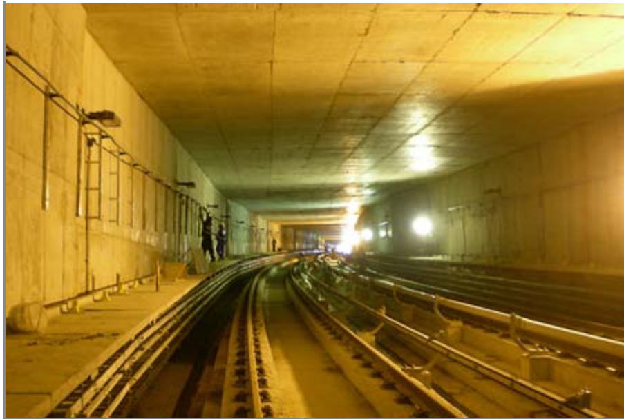
Internal view of the tunnel after the PENETRON treatment.
