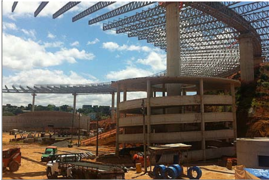
View of the roof structure.
